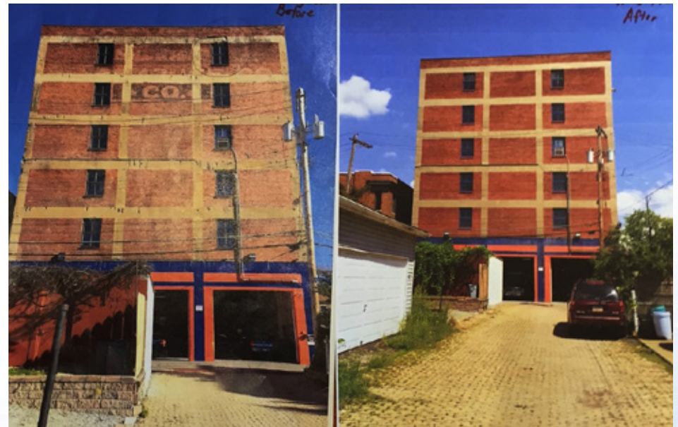
Bloomfield before and after masonry repairs.
