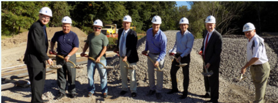
L-R: Jeff Michelson, Desmone Architects; Bob Kelly, Investor; Eric Kulikowski, Investor; John Clingan, First Commonwealth Bank; Bill Krahe, Guardian Storage Development Partner; Steven Cohen, Guardian Storage President; Grant Scott, Meyer Unkovic & Scott Attorneys at Law; Gus Marquart, Bridges Construction
